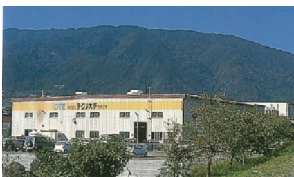
OTE Technological Engineering Corporation, Gifu Plant
