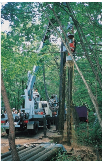
Water Well Drilling water wells down to 50-250m in depth.
